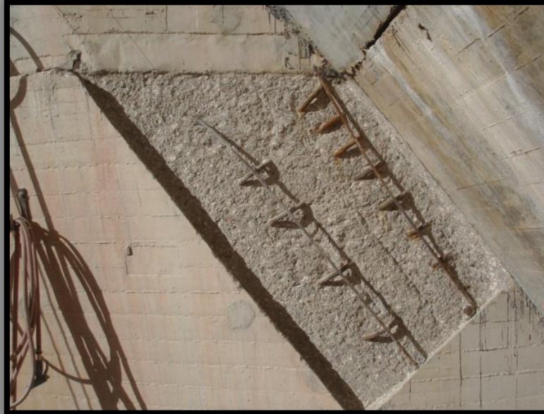
Removal of deteriorated concrete
