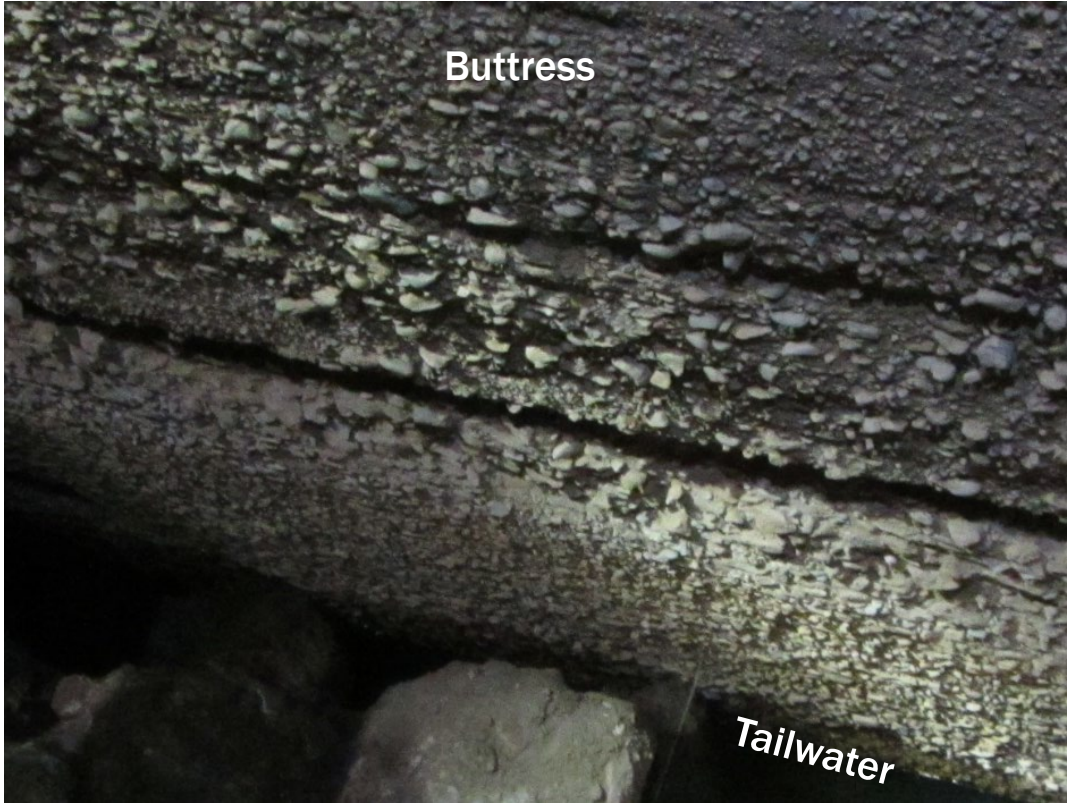
Deteriorated Concrete
