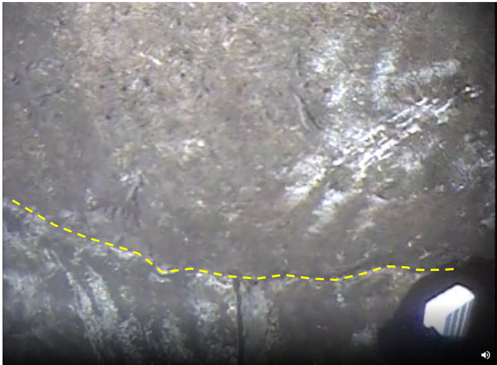
Upstream Slab Crack/Feature
