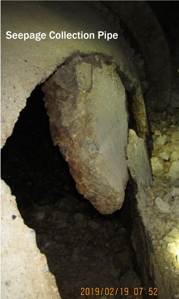
Collapsed Concrete Pipe
