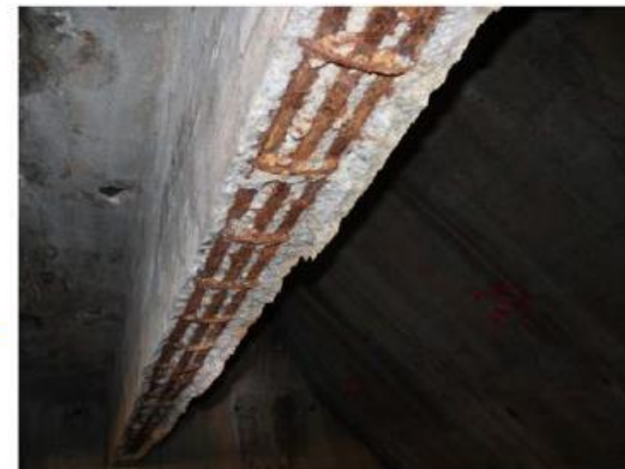
Photo 1: 8/9 Walkway Beam Delamination and Exposed Reinforcement
