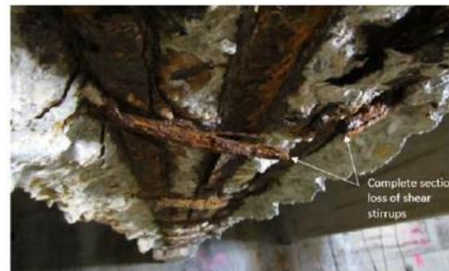
Photo 2: 8/9 Walkway Beam Delamination and Exposed Reinforcement
