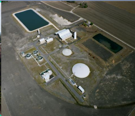
East Williamson County Water System
