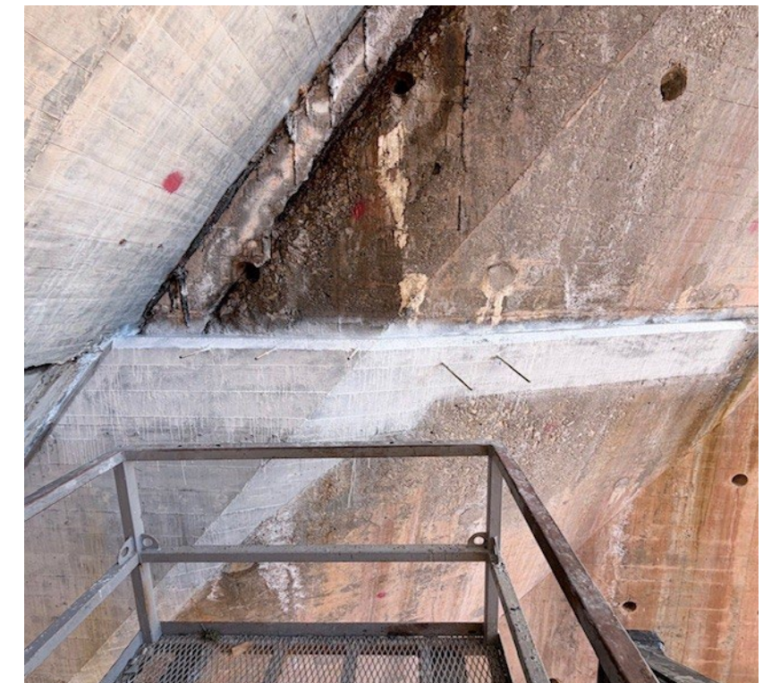
Bay 31 Buttress 31 Corbel Repair
