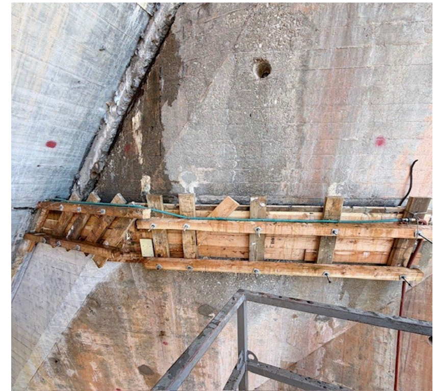
Bay 31 Buttress 31 Corbel Repair
