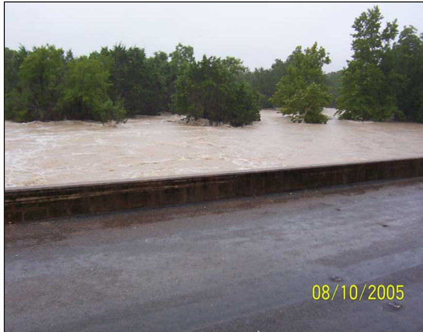
Trimmier Creek out of its banks on 10 th August 2005
