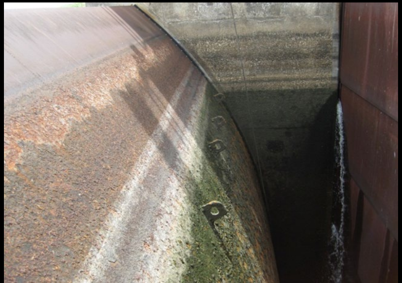
Pictured above: Upstream side of one spillway Tainter Gate at Sterling C. Robertson Dam
