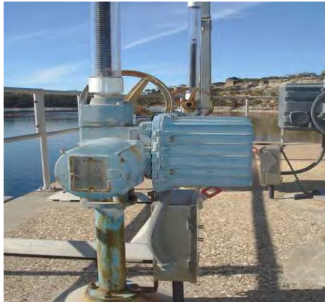
Pictured above: Existing Gate Actuator for Operating Pier at Morris Sheppard Dam.
