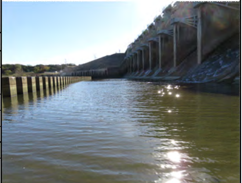
Pictured above: Hearth (facing south) at De Cordova Bend Dam
