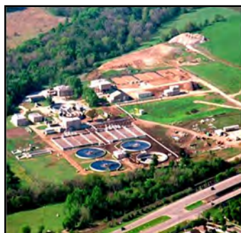
Brushy Creek Regional Wastewater System
