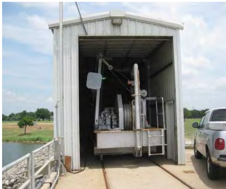
Pictured above: Existing North Hoist Trolley on DeCordova Bend Dam
