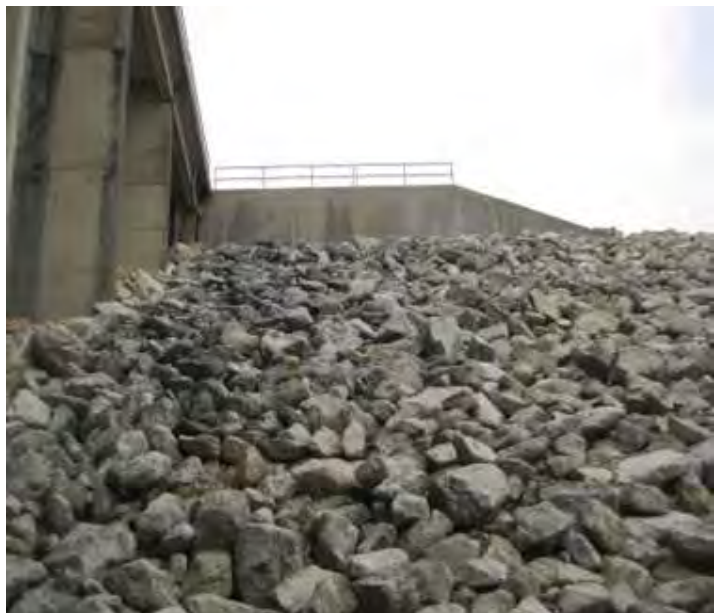
Pictured above: North, downstream embankment retaining wall
