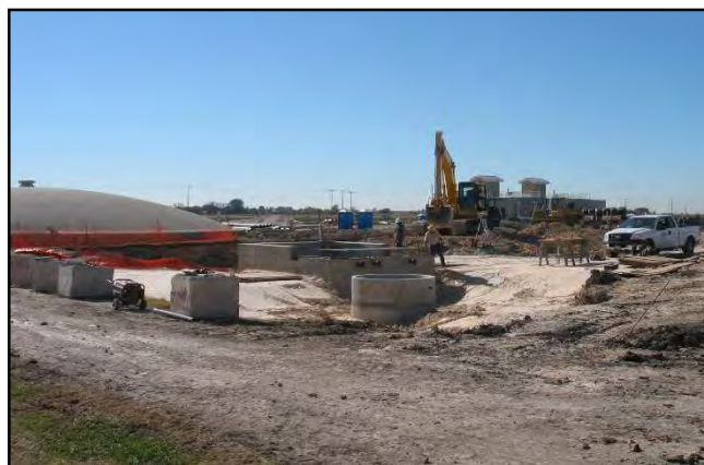
East Williamson County Plant Expansion
