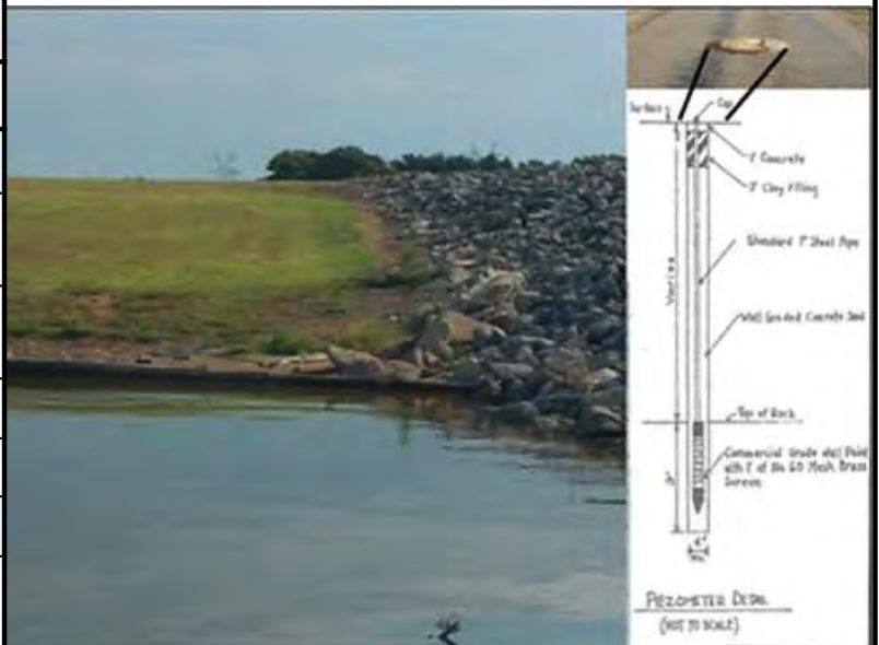
Pictured above: Lake Granbury South Embankment
