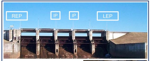
BRA owns and operates Sterling C. Robertson Dam (SCR), which is located in Leon and Robertson Counties. SCR Dam, which forms Lake Limestone Reservoir was completed in 1978. The low flow facilities are located inside the right-end pier (REP), left-end pier (LEP), and intermediate piers (IP). The purpose of the low flow facilities is to release water at rates below 450 cubic feet/second.
