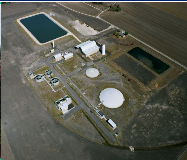
East Williamson County Water System
