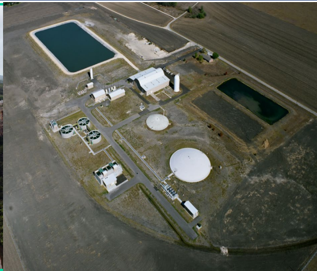
East Williamson County Water System
